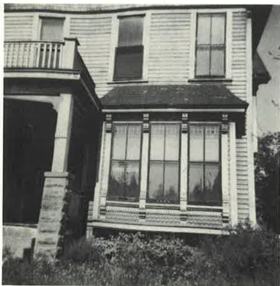
PARSONAGE 2812 West Wisconsin Avenue
